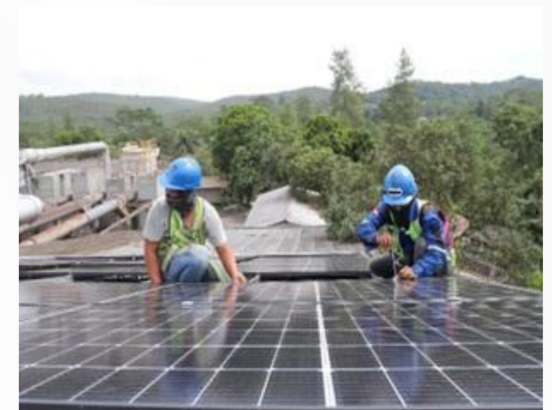
Solar Panel Installation
